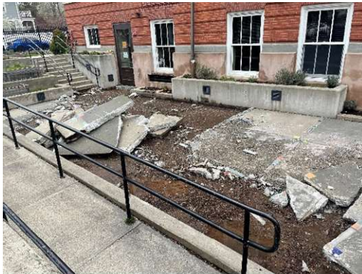
May 2022 project managed by GTS for NHPS Sidewalk at Hooker Elementary
